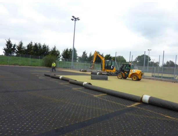
Rolling up carpet – limiting damage during process
